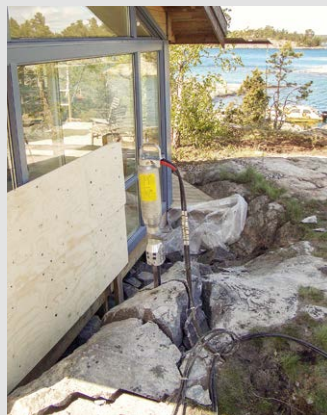
Demolition of rock and natural stone
